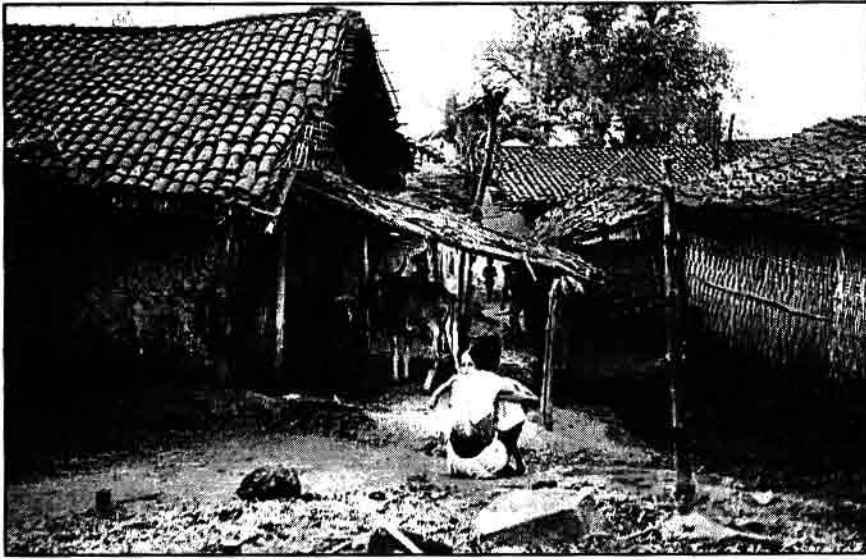
Fig. 10. Houses of Pahavadi. Note the use of mud, wood and hand-made roof tiles
