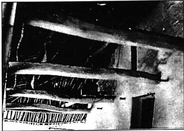
Fig. 5. Tiles atop wooden beams
